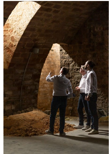
An exceptional vaulted room for hosting events will be created from part of the former wine cellar.
