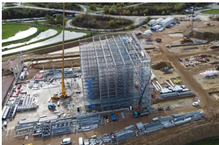
Construction site Progroup Board PW15, date: October 2022 Petersberg, Rhineland-Palatinate, Germany
