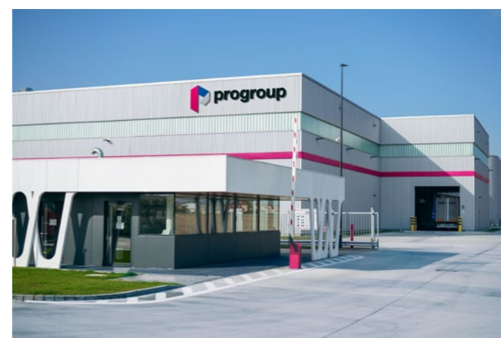
Progroup Board PW10 plant Trzcinica, Poland
