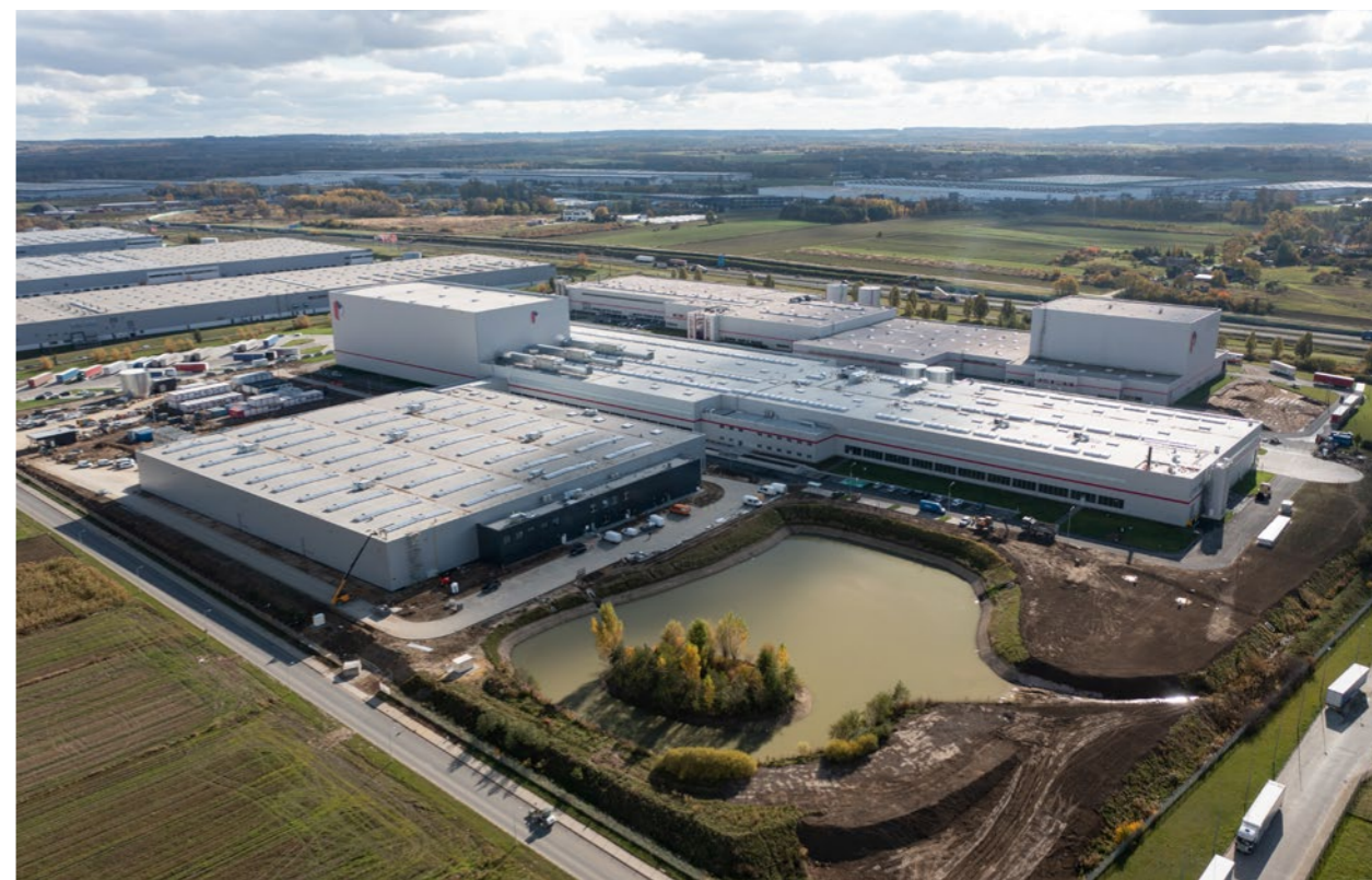
Construction site Progroup Board PW14, date: October 2022 Stryków, Poland
