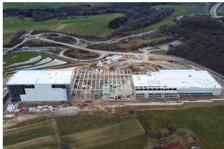
Construction site Progroup Board PW15 Petersberg, Germany
