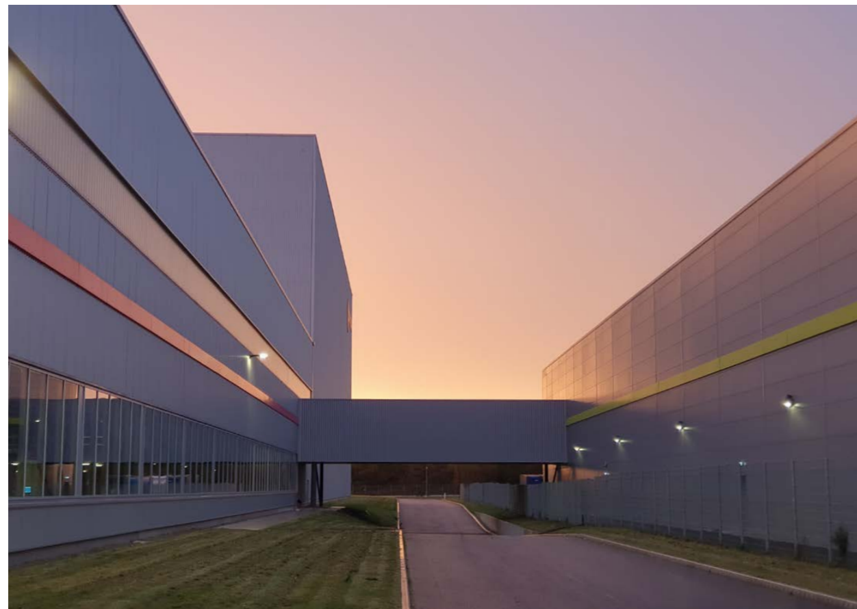
Transport bridge PW12 Ellesmere Port, United Kingdom
